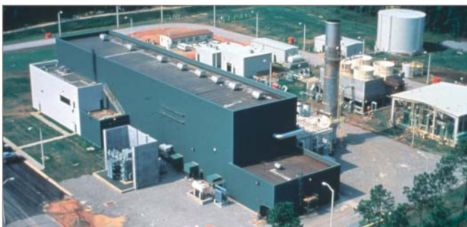
Fig. 6. The 110 MW, 26 h compressed-air energy storage plant at Macintosh, Alabama—one of only two in the world (source: EPRI)
