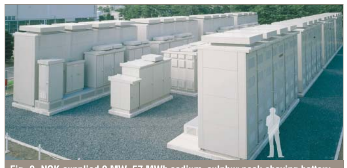
Fig. 9. NGK-supplied 9 MW, 57 MWh sodium–sulphur peak-shaving battery for Hitachi—one of the largest energy storage batteries in the world (source: Hitachi/NGK)
