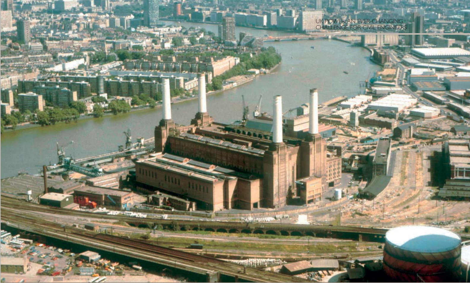
Fig. 1. The 509 MW Battersea power station in London started producing electricity in 1933 with 69 MW generating sets
